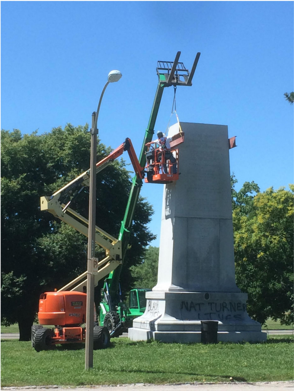
Figure 2. Removal of the Confederate Memorial’s top section, on June 19, 2017.
